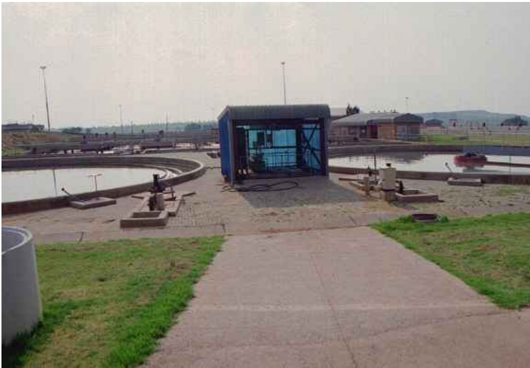
Figure A-6 - Secondary Settling Tank
