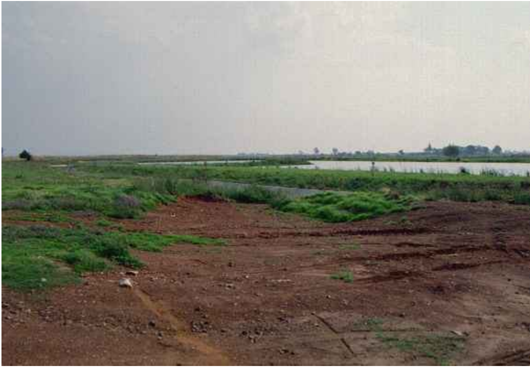
Figure A-9 - Maturation pond provides a degree of polishing of the treated effluent discharged from the mechanical treatment process
