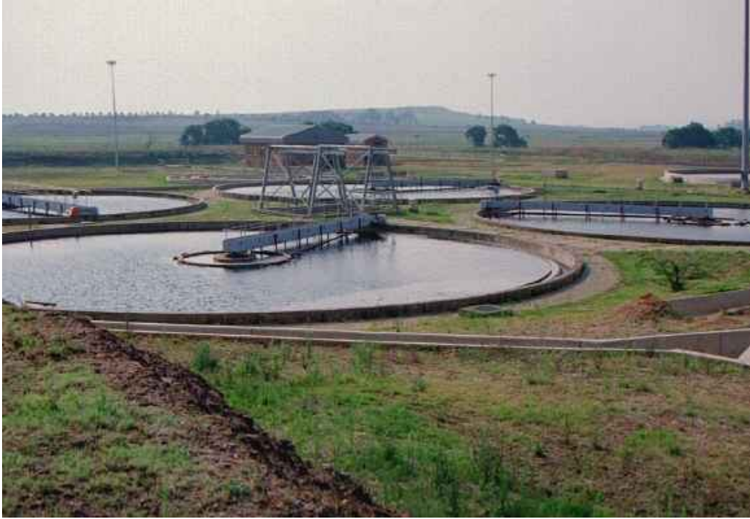
Figure A-8 – Secondary settling tanks used to separate solid particles from water
