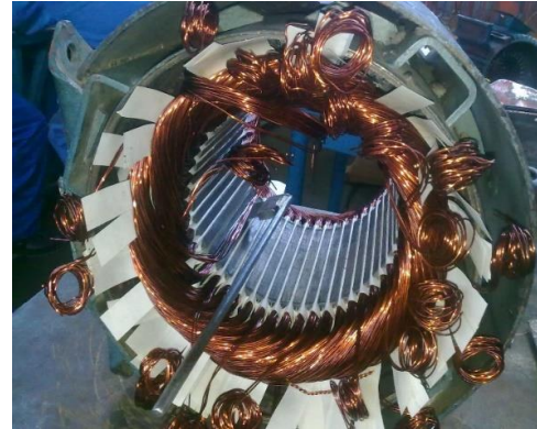
Fig. 3: Traditional rewinding of an induction motor stator with distributed windings [32].
